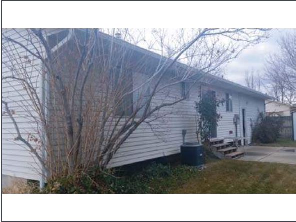
Structure, Rear, Structure 1, Main Dwelling
