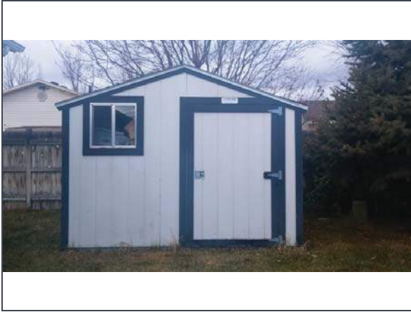
Structure, Front, Structure 2, Toolshed
