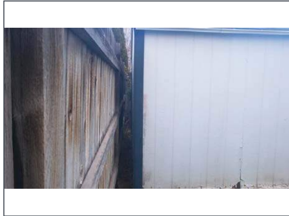
Structure, Rear, Structure 2, Toolshed
