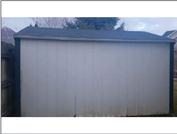
Structure, Left, Structure 2, Toolshed
