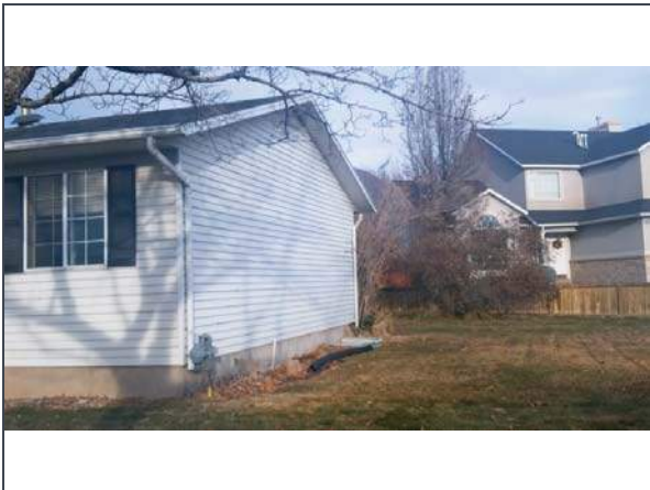
Structure, Right, Structure 1, Main Dwelling
