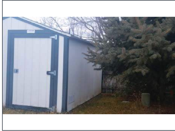
Structure, Right, Structure 2, Toolshed
