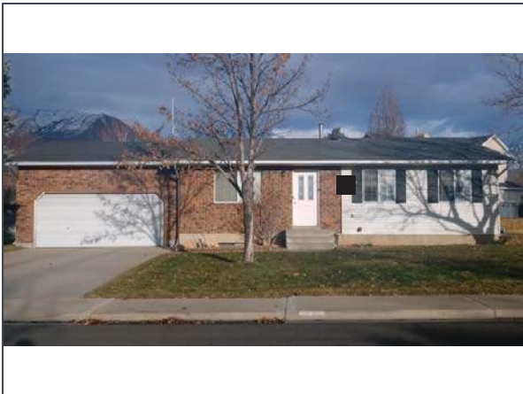
Structure, Front, Structure 1, Main Dwelling
