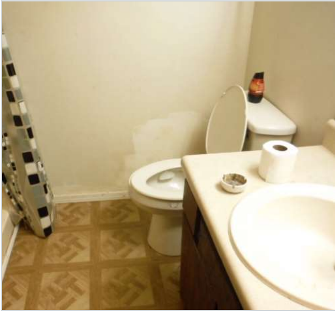
Subject 5557 Windwood Road View Bathroom Comment "5553 Windwood - Bath"
